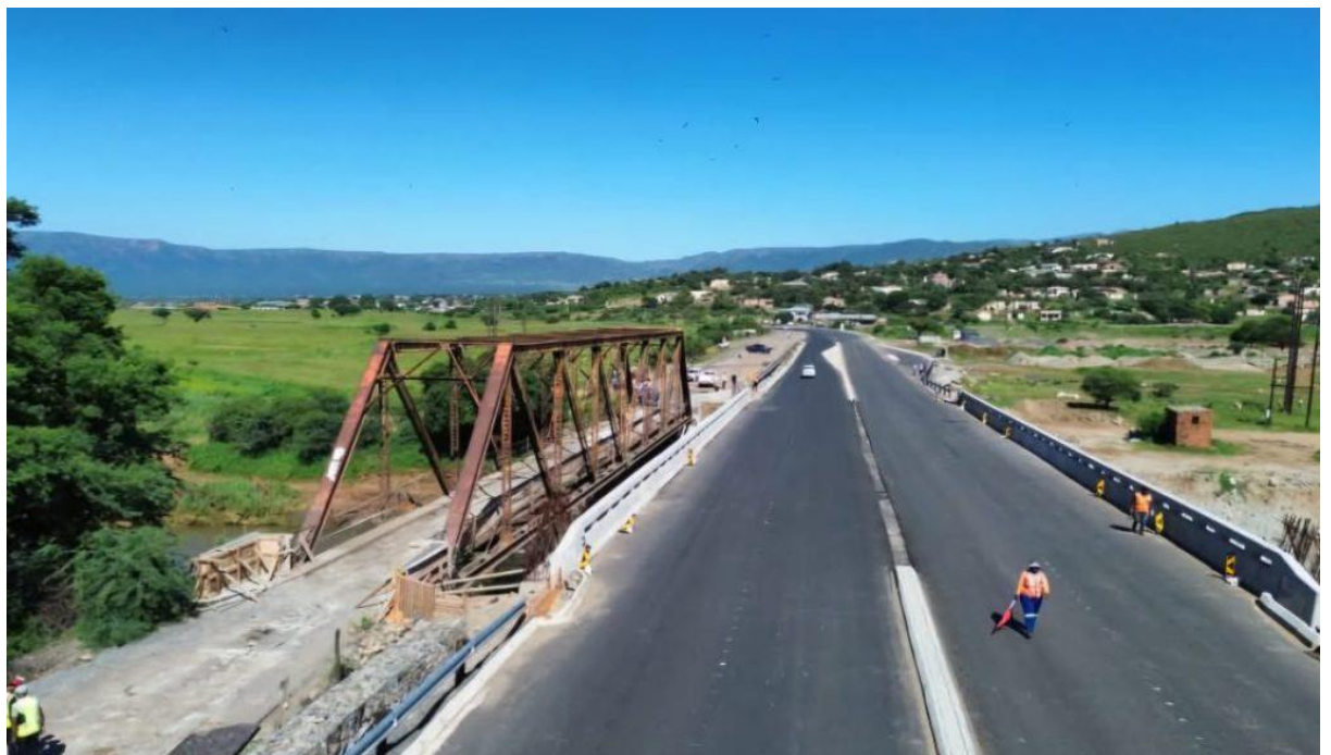
Figure 5.2: Road and Bridge Construction Collaboration Project
