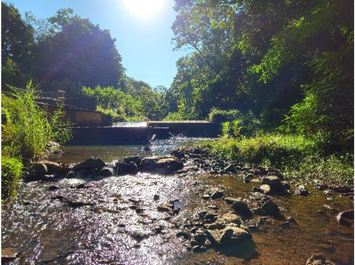
A weir along the Lutandwa River, a tributary of the Luvuvhu River. Photo by Samkelisiwe T Themba
